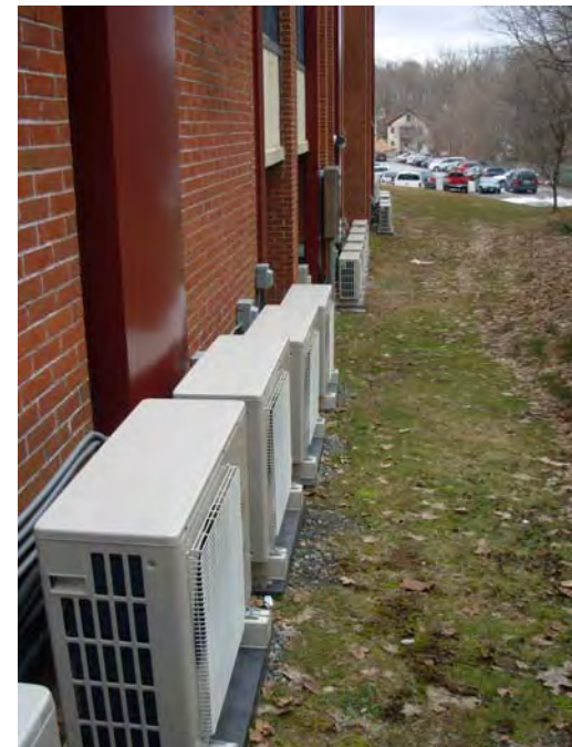
20. Heat pump HVAC system exterior condensers, serving each apartment
