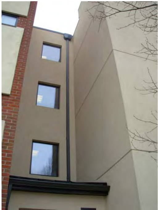
5. EIFS finished surfaces at elevator tower addition
