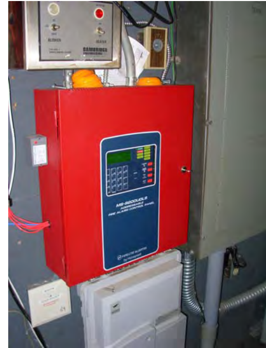
14. Recently updated fire detection - monitoring system
