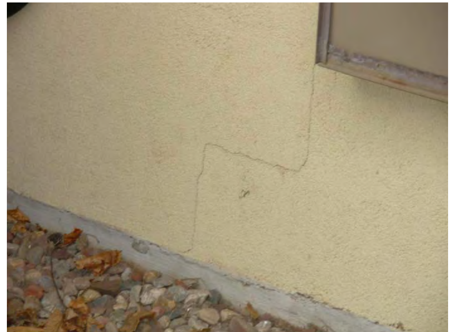
4. Spot step cracking at stucco covered surfaces
