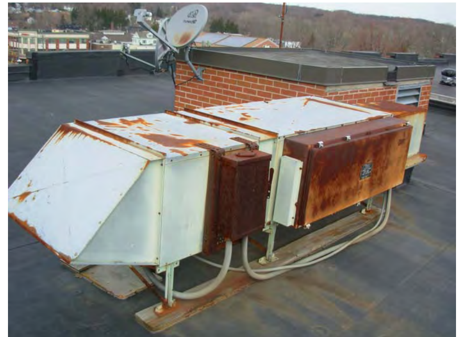
12. Rooftop air handling unit, to replace
