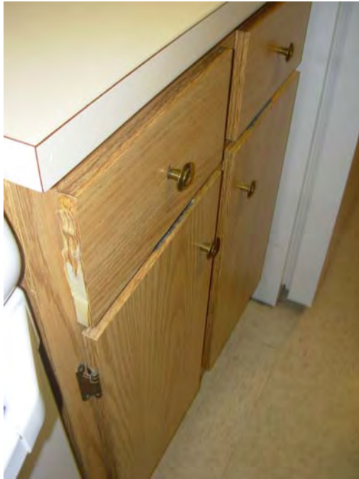
17. Spot delamination of kitchen cabinetry
