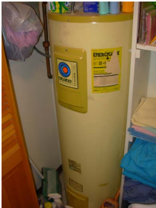
19. Typical unit domestic hot water tank
